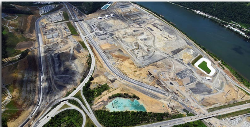
Site of Shell's pending ethane cracker
