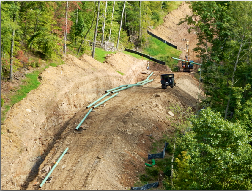
Pipeline land impacts
